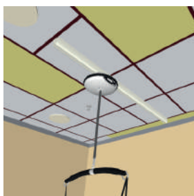
75mm track used with suspended ceiling.
